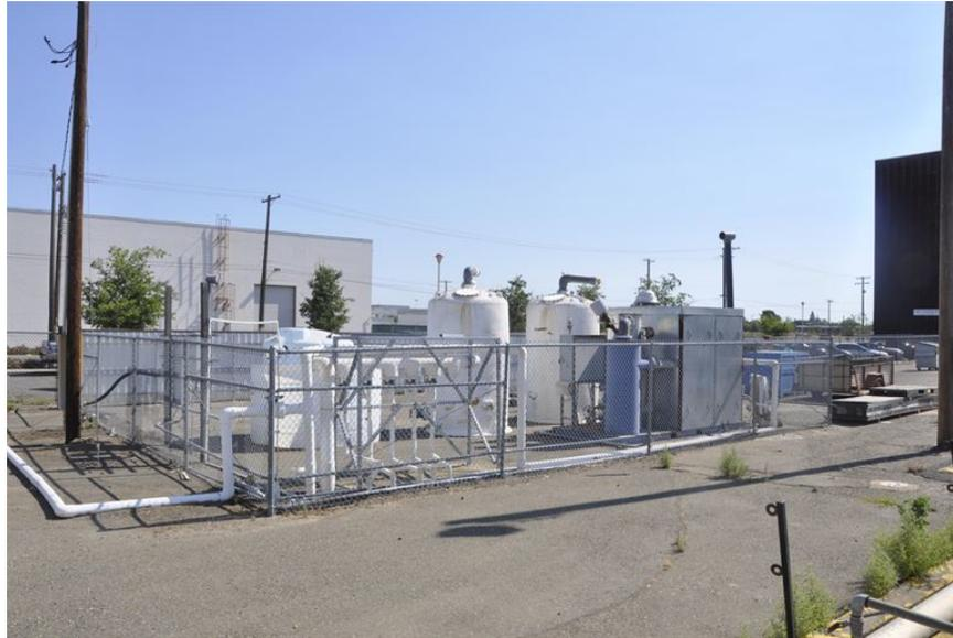
Figure 1: Soil Vapor Extraction
